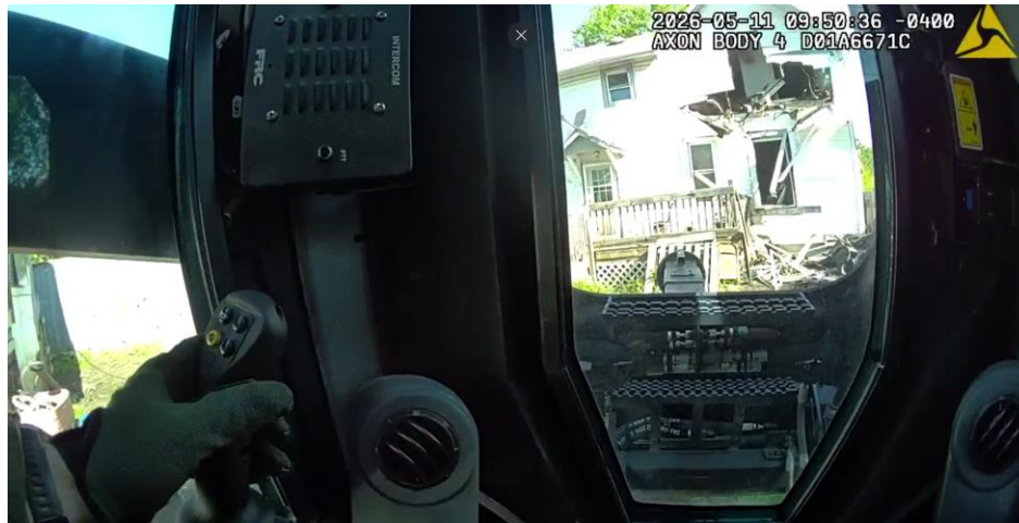
Figure 6: Damage to Rear Second Floor Window
